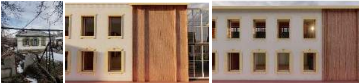
Figure 5 – Interpreted elements of façade
