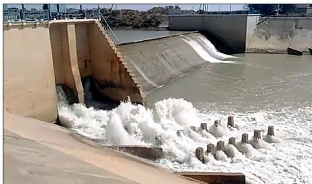
Fig. 1. Overflow surface of the Karaspan hydraulic complex
